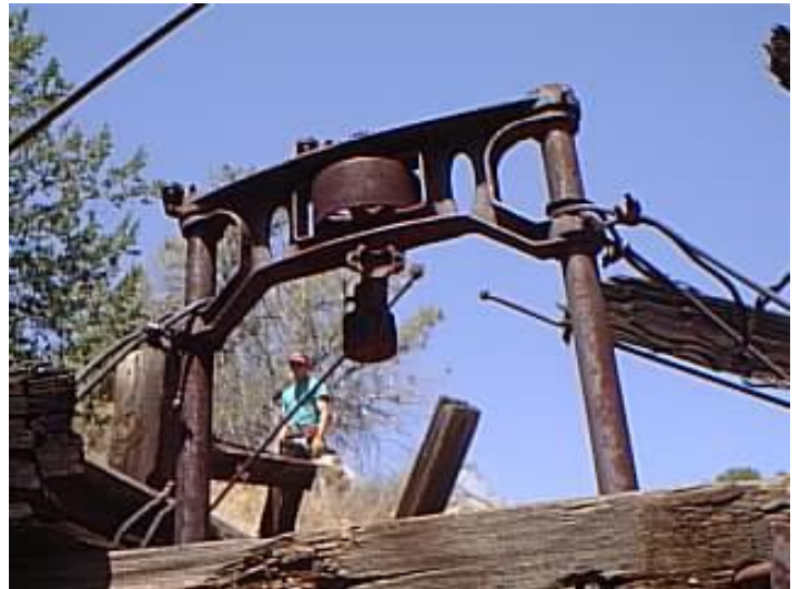
Pulley and shaft.
